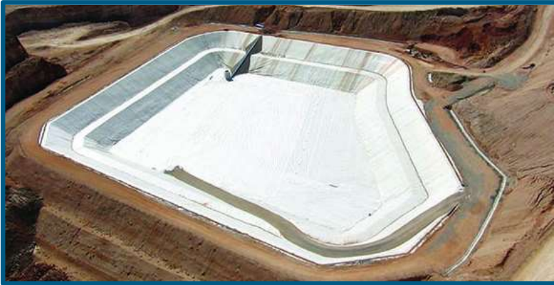
Landfill Liners / Waste Encapsulation
