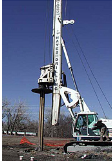
Modified Excavator Drill Rig
