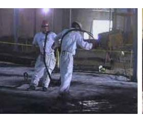
LOWE'S in Ithaca, NY – A total of 115,000 square feet of the LIQUID BOOT® Gas Vapor Barrier was installed, as specified by ElectroMech Engineering, to protect the structure, which was situated on a former landfill site, from the threat of methane vapor instrusion.
