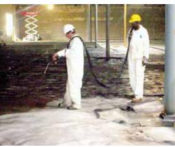
LOWE'S in Ocean Township, NJ – A total of 130,000 square feet of the LIQUID BOOT® Gas Vapor Barrier was installed by CETCO Certified Installer, Edgeboro International,to protect the structure, which was situated on a former landfill site, from the threat of methane vapor instrusion
