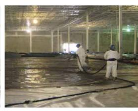
LOWE'S in Patterson, NJ – CETCO Certified Installer, EAI, Inc. installed a total of 145,000 square feet of the LIQUID BOOT® Gas Vapor Barrier, as specified by the engineer, CH2M Hill, in order to protect the structure from the potential threat of residual VOC vapors that were detected in the soil.
