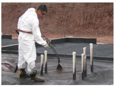
In addition to superior chemical resistance performance, LIQUID BOOT® LT sprayapplication effectively seals penetrations, footings, grade beams and other irregular surfaces that are considered critical vapor intrusion pathways.
