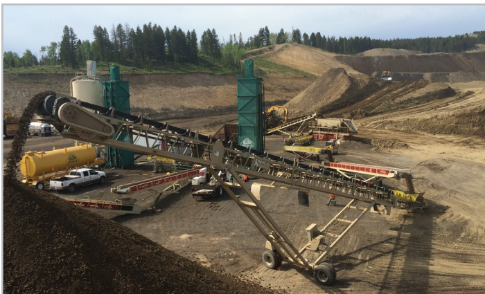
Photo 4. – Placement of mixed soil and bentonite.
