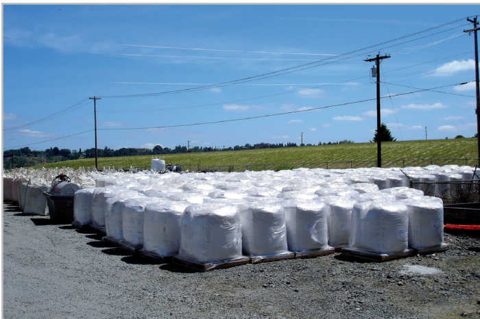
Photo 2. – Supersacks of Volclay delivered to a job site are ready to be placed in a grid pattern to ensure proper application rates.
