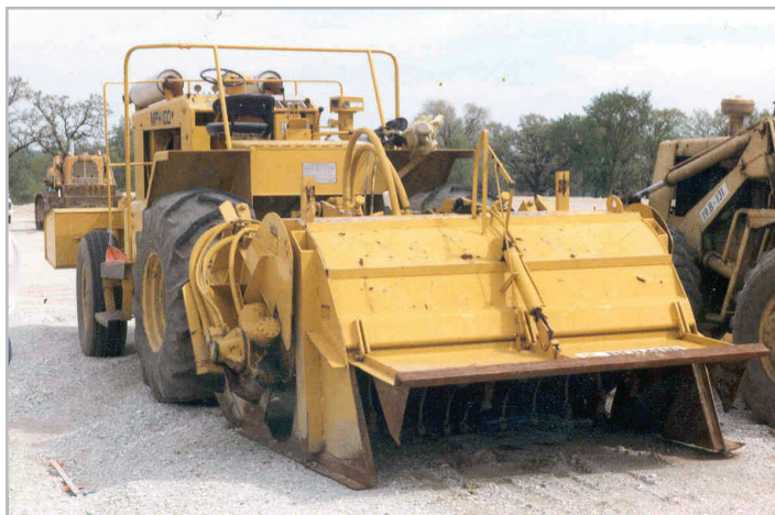
Photo 1. – A Bomag “recycler,” normally used to recycle asphalt pavement, does an excellent job of mixing soil and Volclay.
