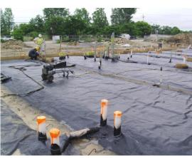
Images left to right: GEOVENT™ trenchless gas venting system being installed directly on the subgrade; LIQUID BOOT® vapor barrier conforms to irregular surfaces and can be applied in the most challenging conditions; LIQUID BOOT® spray-application effectively and effortlessly seals around crucial areas, such as pipe penetrations.
