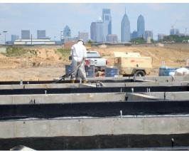
Images left to right: BASEFABRIC™ T-60 provides a uniform substrate to spray the LIQUID BOOT® vapor barrier; the spray-application fully adheres to irregular surfaces, allowing for ease of installation, labor savings, and a gas-tight and seamless barrier; LIQUID BOOT® vapor barrier being installed by a certified applicator on each of the building footprints.
