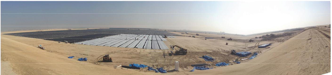
CETCO developed a membrane-laminated RESISTEX® GCL for the containment of caustic liquor from the bauxite refining process at the ALCOA-Maaden's integrated aluminum project in Ras Al Khair, Saudi Arabia. The 0.5 mm membrane component of the GCL was fully welded, with the GCL seams constructed in traditional overlapped fashion.
