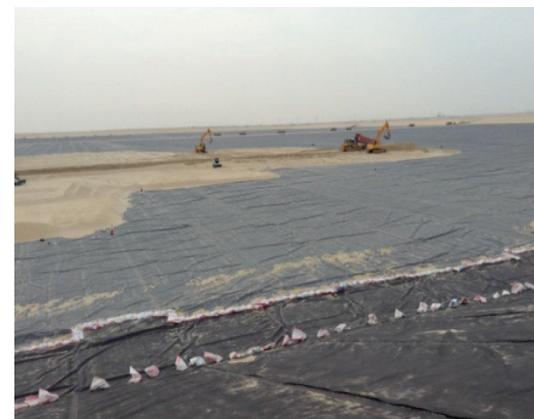
CETCO developed a membrane-laminated RESISTEX® GCL for the containment of caustic liquor from the bauxite refining process at the ALCOA-Maaden's integrated aluminum project in Ras Al Khair, Saudi Arabia. The 0.5 mm membrane component of the GCL was fully welded, with the GCL seams constructed in traditional overlapped fashion.
