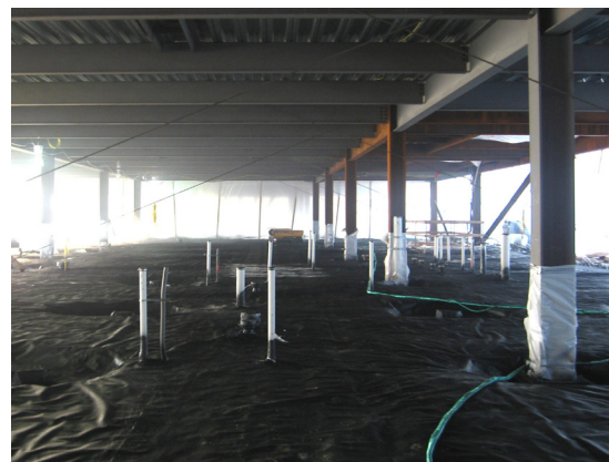
Left to right: installation of the GEOVENT™ sub slab venting system; spray-application allows for quick and air-tight seal around all penetrations and irregularities to save considerable time; installed spray-applied vapor membrane attaches to the piles themselves and conforms to the haunch.
