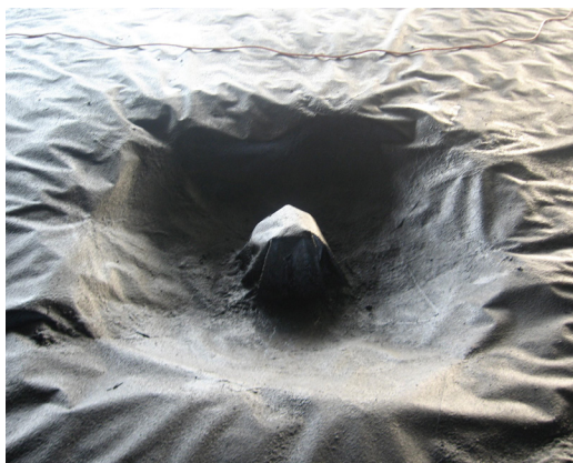
Left to right: installation of the GEOVENT™ sub slab venting system; spray-application allows for quick and air-tight seal around all penetrations and irregularities to save considerable time; installed spray-applied vapor membrane attaches to the piles themselves and conforms to the haunch.
