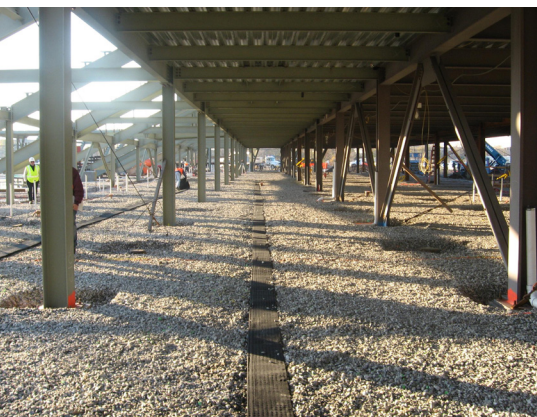
Left to right: installation of the GEOVENT™ sub slab venting system; spray-application allows for quick and air-tight seal around all penetrations and irregularities to save considerable time; installed spray-applied vapor membrane attaches to the piles themselves and conforms to the haunch.
