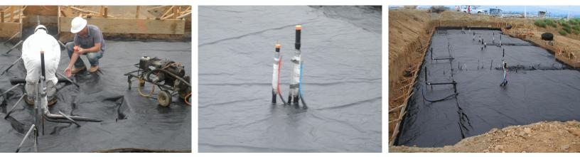
A CETCO-pioneered smoke test (image on left) was performed on the LIQUID BOOT® vapor barrier after it was installed to ensure a quality and gas tight installlation.
