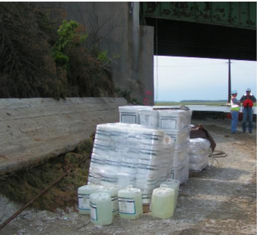
Mixing SHORE PAC polymer with the marina's water allowed for desired viscosities and an economical solution to trucking in freshwater. Even though the intrusion of saltwater into the drilled shafts could not be stopped, consistent maintainable viscosities were achievable using the freshwater for mix water.
