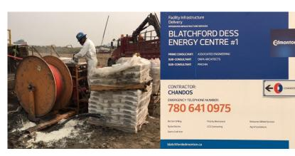
In May 2018, a drilling contractor started the installation of 570 (6" diameter x 500ft deep) geothermal boreholes in Edmonton, AB, Canada. The project at the former Edmonton Municipal Airport started with 2-rigs drilling in a formation of clay, silt, and coal seams. It increased to multiple rigs before the successful completion in October 2018. The grout development started prior to the first hole being drilled onsite.
