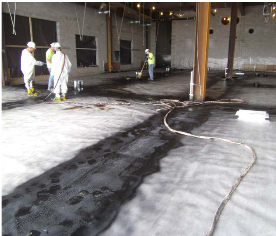
Utilizing CETCO's gas vapour mitigation system and Geovent allowed the client to develop this larger brownfield site.
