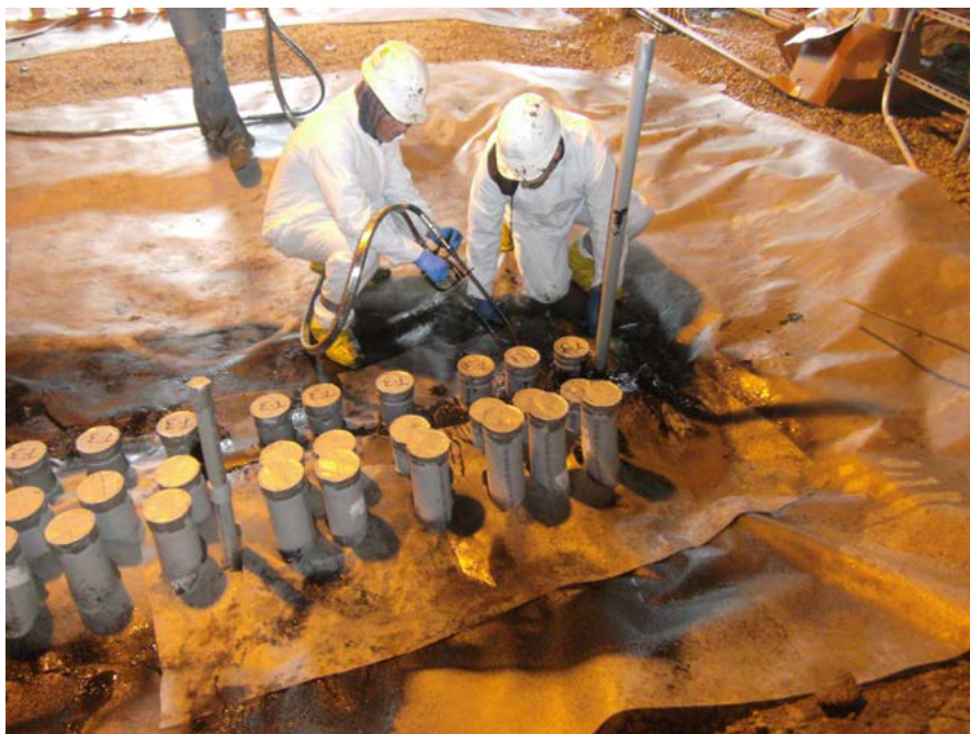
Applying the Liquid Boot vapour intrusion barrier system.
