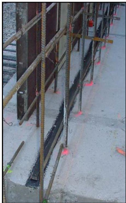
Figure 1. Properly installed Waterstop-RX prior to concrete encapsulation.
