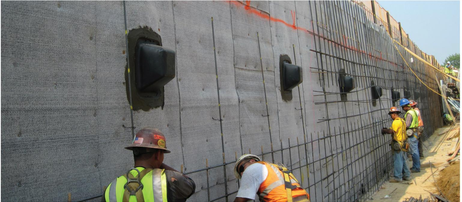
Install VOLTEX® GB-500 waterproofing membrane composite with geotextile side against the cast-in-place concrete foundation walls prior to backfilling. VOLTEX® GB-500 waterproofing membrane composite may be applied as soon as the forms are removed. It is not necessary to wait for the concrete to completely cure. Use VOLTEX® GB-500 waterproofing membrane composite with concrete cast with conventional forms that produce smooth surface.
