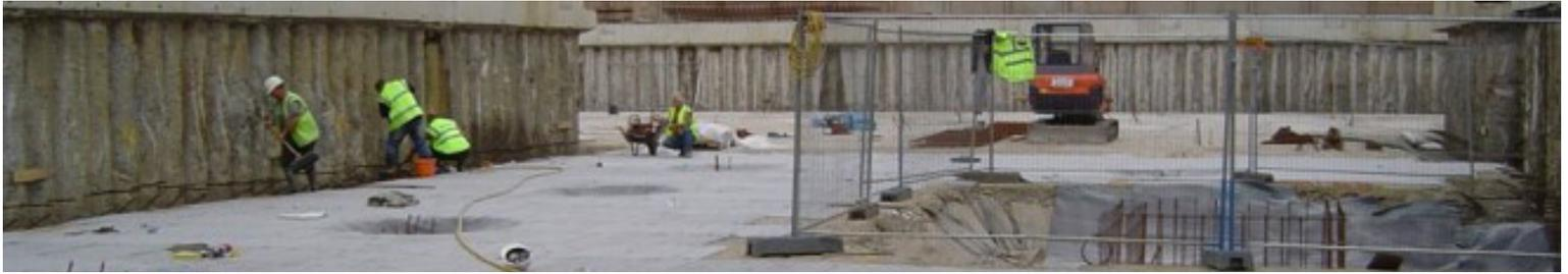
VOLTEX® GB-500 waterproofing membrane composite is designed for below-ground waterproofing applications where the product is properly confined. VOLTEX® GB-500 waterproofing membrane composite and accessory products should not be installed in standing water or over ice. If ground water contains strong acids, alkali's, or is of a conductivity of 6,000  $\mu\text{mhos/cm}$  or greater, water samples should be submitted to the manufacturer for compatibility testing.
