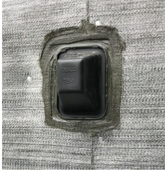
PHOTO 3: TB-BOOT OVER (HYDROSTATIC)
