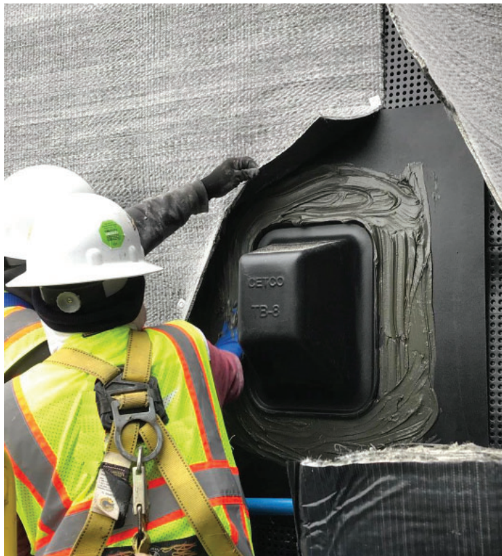
PHOTO 4: TB-BOOT (NON-HYDROSTATIC)
