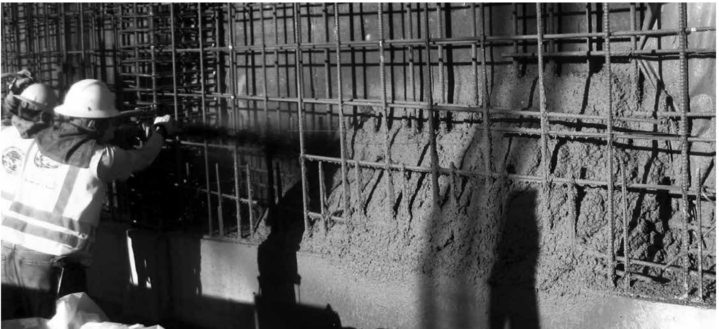
PHOTO 2: SHOTCRETE FOUNDATION WALL
