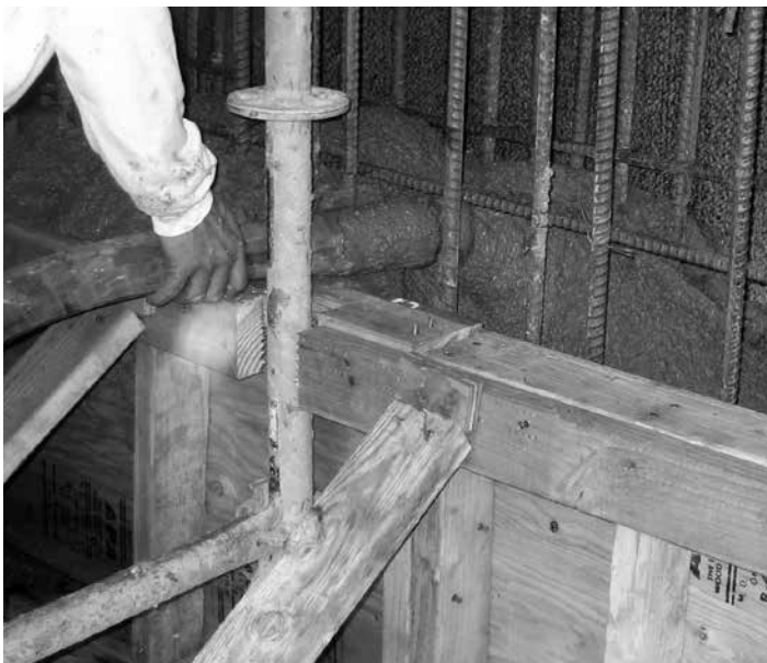
Photo H3-3: SHOTCRETE PLACEMENT IN KICKER FORM
