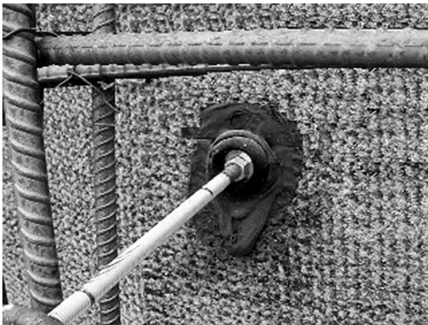
PHOTO 4: REBAR ANCHORAGE DETAILING
