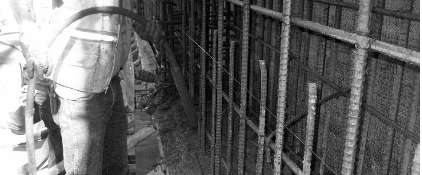
PHOTO 1: KICKER FORM AT BASE OF SHOTCRETE WALL
