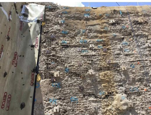
With a geomembrane ten times more impermeable than traditional hydrophilic membranes, the expanding action of ULTRASEAL AB waterproofing membrane swells to seal any small concrete cracks caused by ground settlement or concrete shrinkage.
