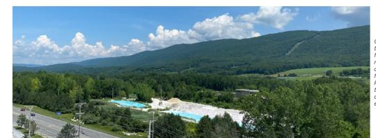
One of our treatment ponds for settling and neutralizing our wastewate from Specialty PCC operations to ensure safe discharge to the environment.
