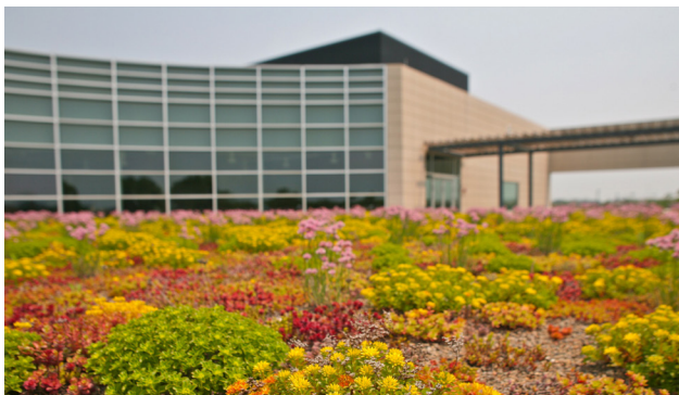
MTI's office and R&D facility in Hoffman Estates, IL is built to LEED standards and includes two green roofs, native planted bioswales and rain-gardens.
