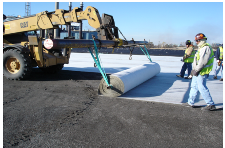
Figure 4-1. Deploying of the liner using core pipe and spreader bar.
