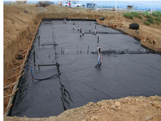
A CETCO-pioneered smoke test (image on left) was performed on the LIQUID BOOT® vapor barrier after it was installed to ensure a quality and gas tight installation.
