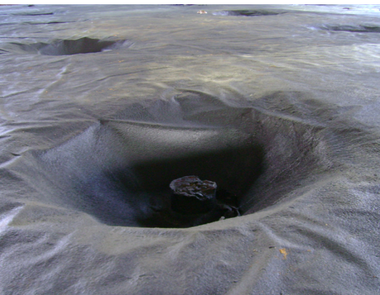
Left to right: The installed spray-applied vapor membrane attaches to the piles and conforms to the haunch; completed vapor membrane is covered with ULTRASHIELD™ P-150 protection material; upon completion, other trade installations can begin.
