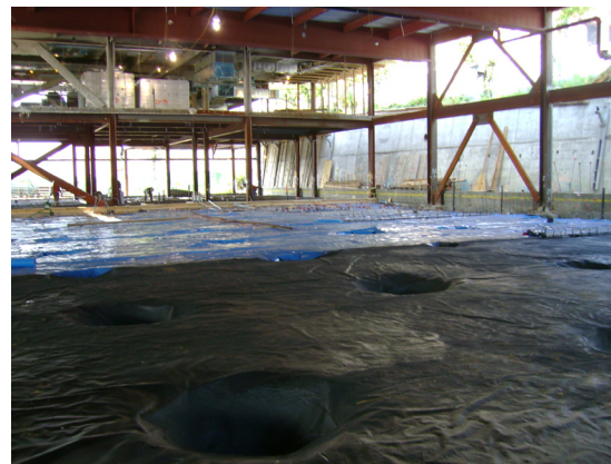
Left to right: The installed spray-applied vapor membrane attaches to the piles and conforms to the haunch; completed vapor membrane is covered with ULTRASHIELD™ P-150 protection material; upon completion, other trade installations can begin.
