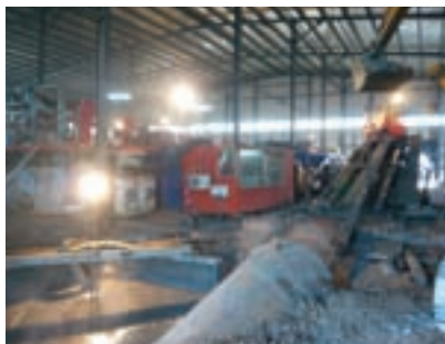
Inside the entrance pit building with HDD rig and mud plant
