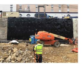
To meet warranty requirements, WATERSTOP-RX® hydrophilic, swelling concrete joint waterstop was used around penetrations and applicable concrete joints. WATERSTOP-RX concrete joint waterstop swells upon hydration to form a positive seal in concrete cold pour joints.
