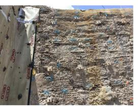
ULTRASEAL AB waterproofing membrane's adhesive layer protects the Active Polymer Core (APC) layer from excessive prehydration during construction allowing it to be installed in all weather conditions and has proven effective in both hydrostatic and non-hydrostatic conditions.
