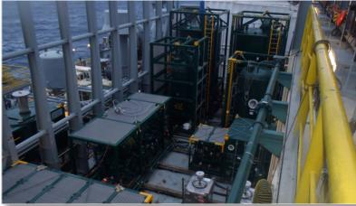
The overboard transfer hose was equipped with a Coast Guard Approved Safety Breakaway Coupling to limit fluid discharge in the event of a boat drive-off. A flare scrubber was installed between the separator and the flare boom to reduce the risk of fluid carryover to the flare. The entire package was designed in accordance with API 14C.
